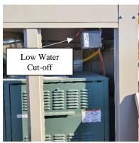
Figure 34 - Low Water Cut-Off Switch
