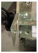
Figure 46 - Flame Roll-Out Switch
