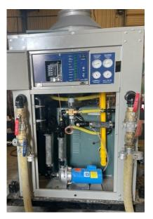
Figure 18 - Primary Circulation Line Connections
