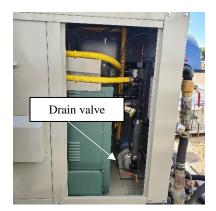
Figure 42 - Circulation Pump/Drain Valve
