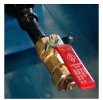
Figure 39 - Drain Valve
