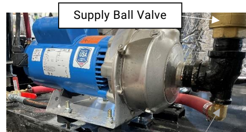
Figure 36 Pump connections
