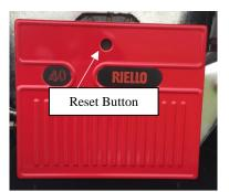
Figure 32 - Burner Reset Button
