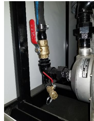
Figure 37 - Fill/Drain Ball Valves (Operating Position)
