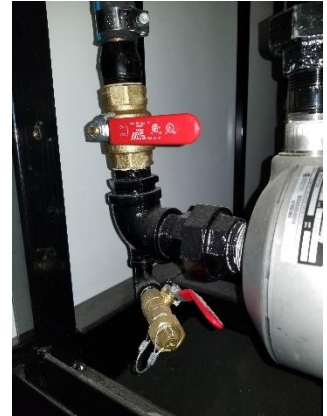
Figure 36 - Fill/Drain Ball Valves (Filling)
