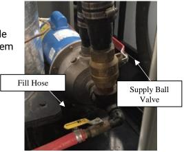
Figure 33 - Pump Connections
