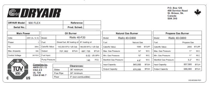
Figure 50 - Water Heater Data & Serial Plate
