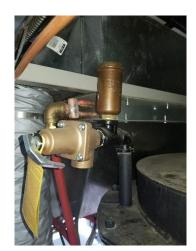
Figure 28 - Automatic Air Vent Valve Cap
