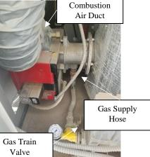
Figure 24 - Propane Gas/Natural Gas Burner Connections
