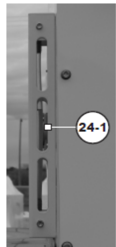
Figure 38-Glycol Level Gauge
