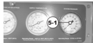
Figure 19-System Pressure Gauge
