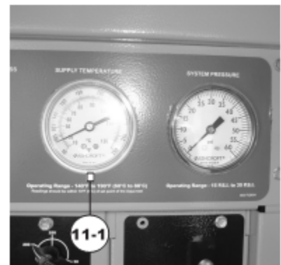
Figure 25-Supply Temperature Gauge
