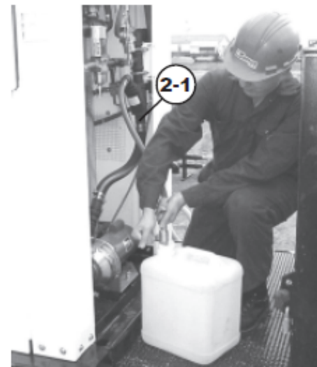
Figure 47-Back Washing Y-Strainer
