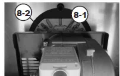
Figure 14-Riello Burner Tube & Mounting Bracket
