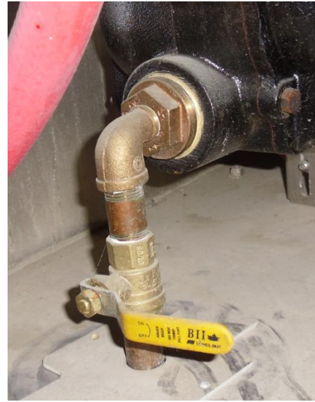
Figure 13 - Condensate Drain Valve
