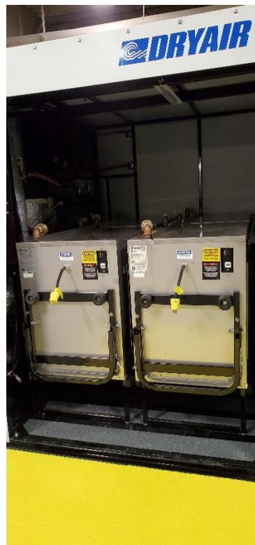
Figure 44 - Storage Bay with 4x 200 HCP Edition Fan Coils
