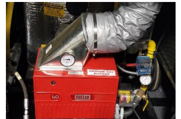
Figure 27 - Propane Gas Burner
