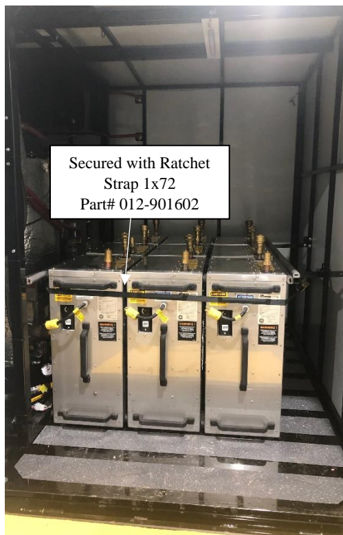
Figure 42 - Storage Bay with 9x 80 Fan Coils
