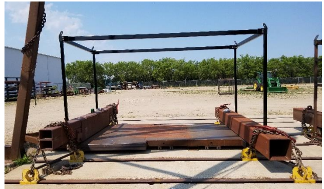
Figure 1. 900-HCP trailer frame and installed lifting frame assembly secured to test bed.
