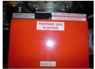
Figure 19 - Propane Gas Burner
