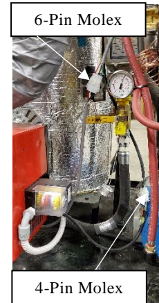
Figure 21 - Electrical Connection
