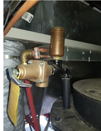
Figure 27 - Automatic Air Vent
