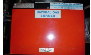
Figure 20 - Natural Gas Burner
