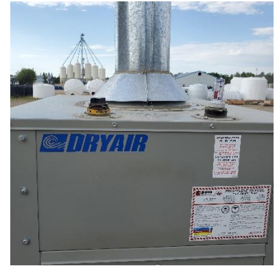
Figure 31 - HTF Fill Cap and Gauge
