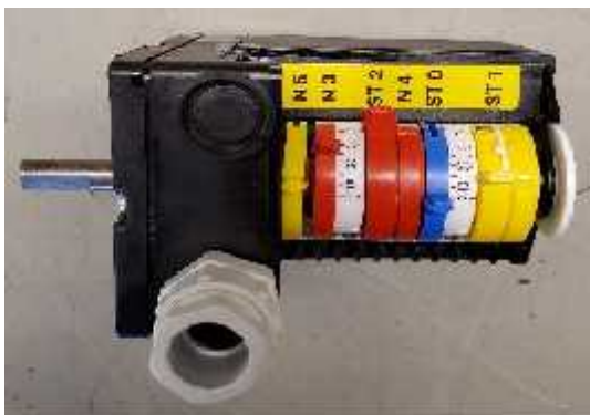
Servo Motor (on side of burner)
