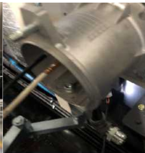
burner swings out remove wires
