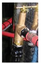
Figure 5-4 Pressure Bypass Valve
