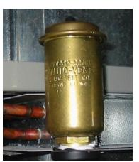
Figure 5-8 Automatic Air Bleed Vent
