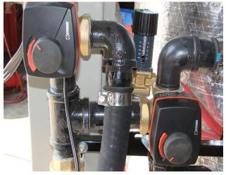
Figure 5-10 Flow Reverser in Default Position
