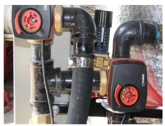
Figure 5-11 Flow Reverser with Indicator Caps Removed
