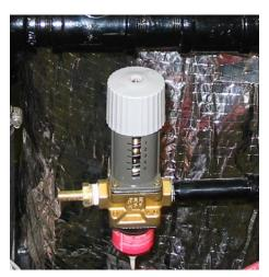
Figure 5-7 Thermostatic Control Valve
