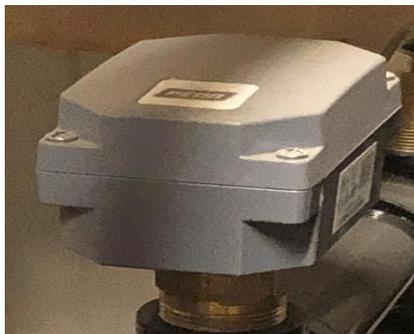
Figure 6-19 Flow Switch model 200/650 GTS
