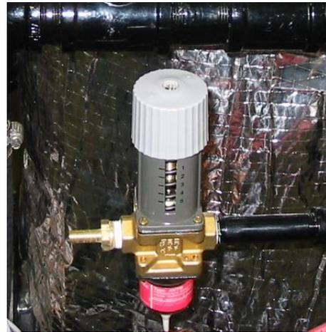
Figure 5-7 Thermostatic Control Valve
