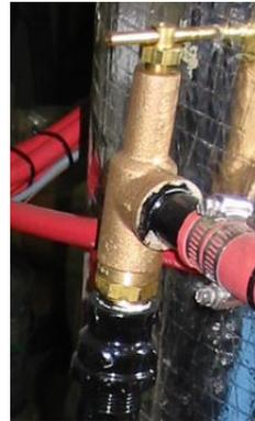
*Figure 5-4 Pressure Bypass Valve*
