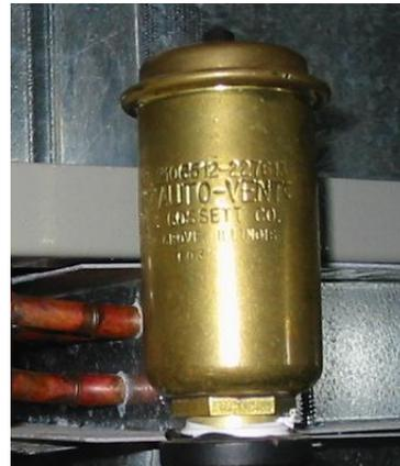
Figure 5-8 Automatic Air Bleed Vent
