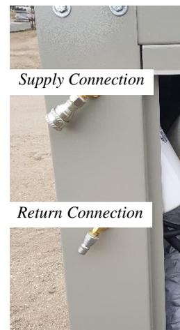
Figure 4-18 External Diesel Connection
