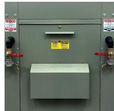
Figure 4-5 Supply & Return Isolation Valves
