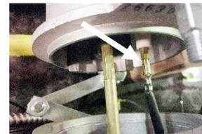
Figure 9-2 Unplug Ignitor Wire
