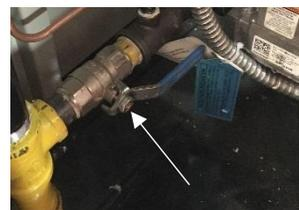
Figure 4-8 Internal gas valve
