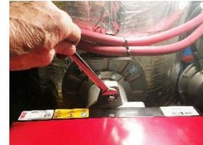
Figure 9-1 Burner Retaining Nut
