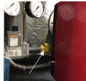
*Figure 8-2 Burner Gas Line Connection*
