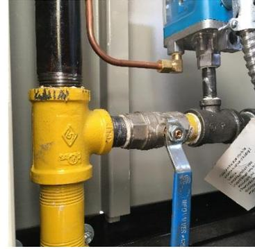
*Figure 6-3 Internal gas valve (closed)*
