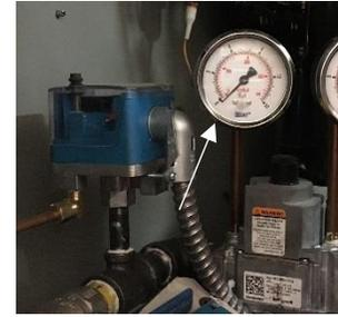
Figure 4-10 Gas supply pressure gauge
