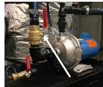
Figure 6-2 Pump Isolation Valve
