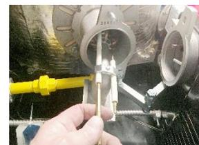
Figure 9-5 Combustion Head Removal
