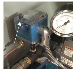
Figure 4-9 Low gas pressure switch reset
