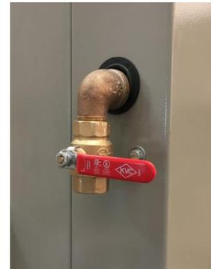
*Figure 6-4 Manual gas valve (closed).*
