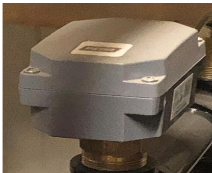
Figure 6-19 Flow Switch model 200/650 GTS
