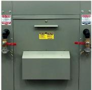
Figure 4-5Supply & Return Isolation Valves
