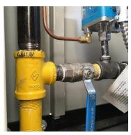
Figure 6-3 Internal gas valve (closed)
