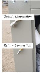
Figure 4-18 External Diesel Connection
