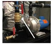
Figure 6-2 Pump Isolation Valve
