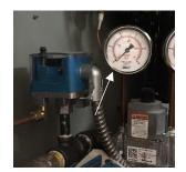
Figure 4-10 Gas supply pressure gauge
