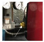
Figure 8-2 Burner Gas Line Connection
