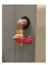
Figure 6-4 Manual gas valve (closed).
