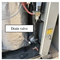
Figure 32 - Circulation Pump/Drain Valve
